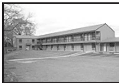
Paved Parking Room Fronts
